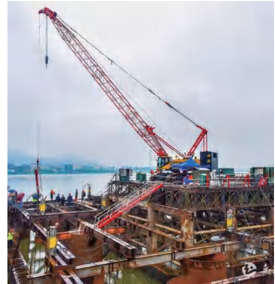
Steel Box Cofferdam with Bottom
