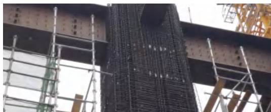
STEEL-CONCRETE COMPOSITE STRUCTURE SYSTEM
