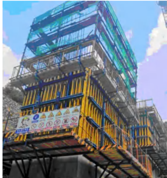
Hoisting Cantilever Support Formwork
