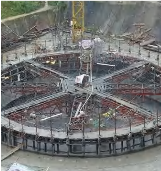
Slip Formwork for Shaft
