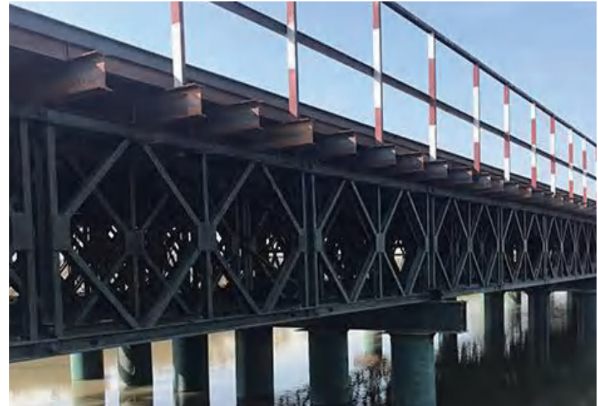
Temporary Steel Bridge
