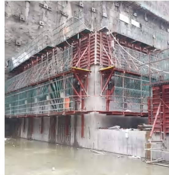
Dam Automatic Lifting Cantilever Formwork
