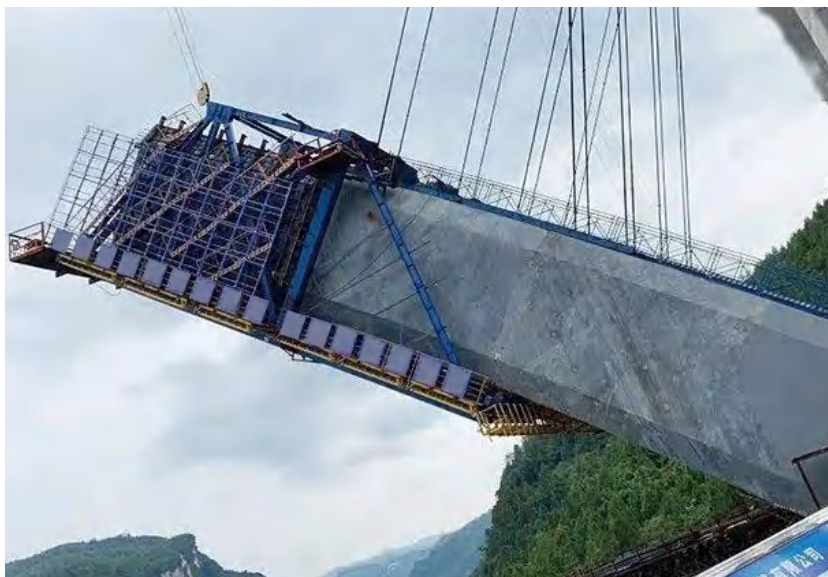
Cantilever Carriage for Arch Bridge
