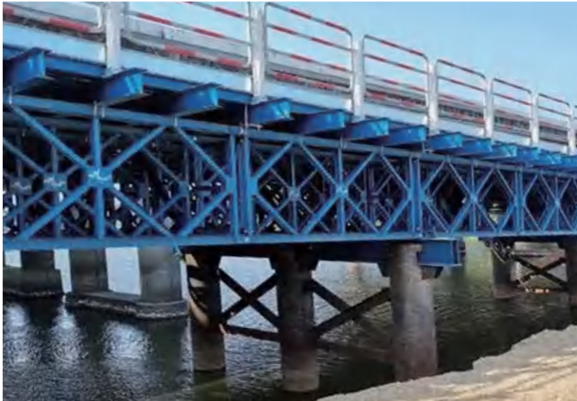
Temporary Steel Bridge
