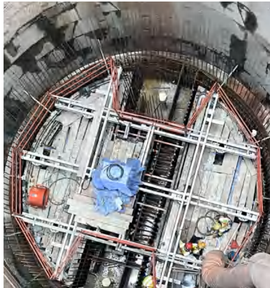
Climbing Formwork for Shaft
