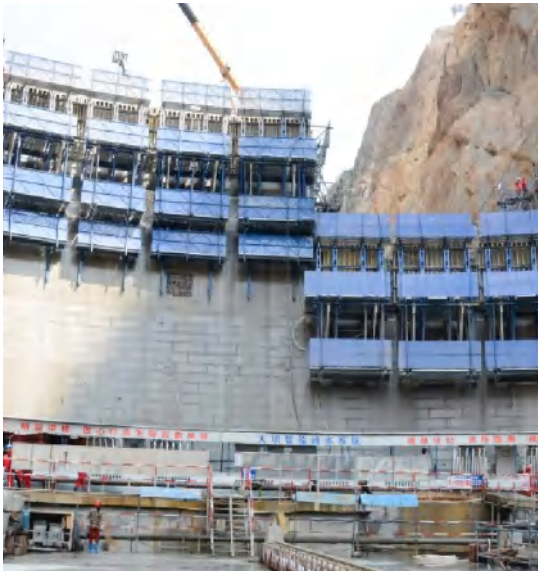
Climbing Formwork for Dam
