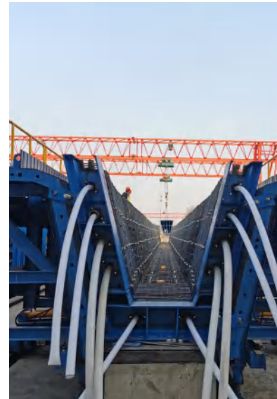
Prefabricated Box Girder (Hydraulic)
