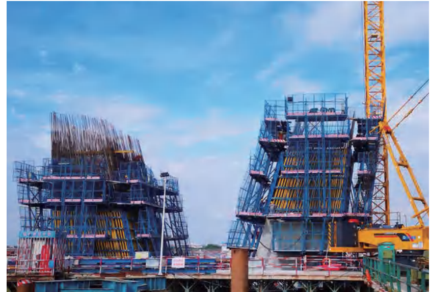
Climbing Formwork for Pier
