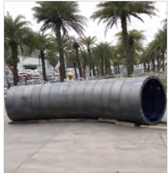
Steel Formwork for Circle Tunnel
