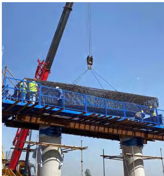
Operation Platform for Bent Cap
